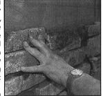
When laying stone, attempt to keep joints a consistent height and width. Normally vertical and horizontal joints should be staggered to prevent long unbroken lines that may draw the eye to a particular area. Semco recommends installing all corner pieces first, alternating short and long lengths as they are stacked.
