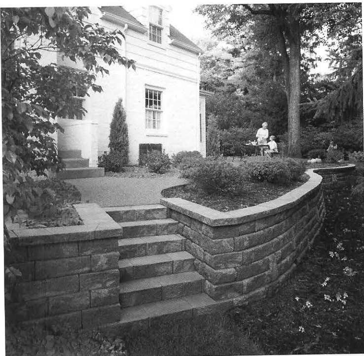
Squaring off the wall next to steps gives a tailored look.
