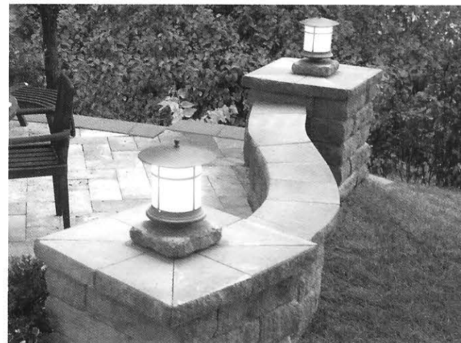
Lights are the perfect way to top off a column. Drill a hole in the coupon and run wiring through the hollow column core.
